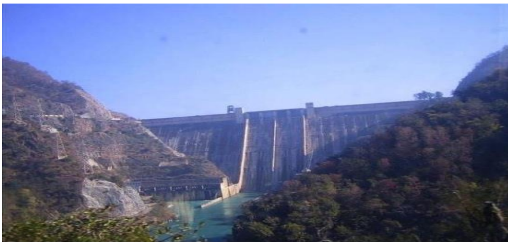
Fig-10 View of Bhakra Dam
