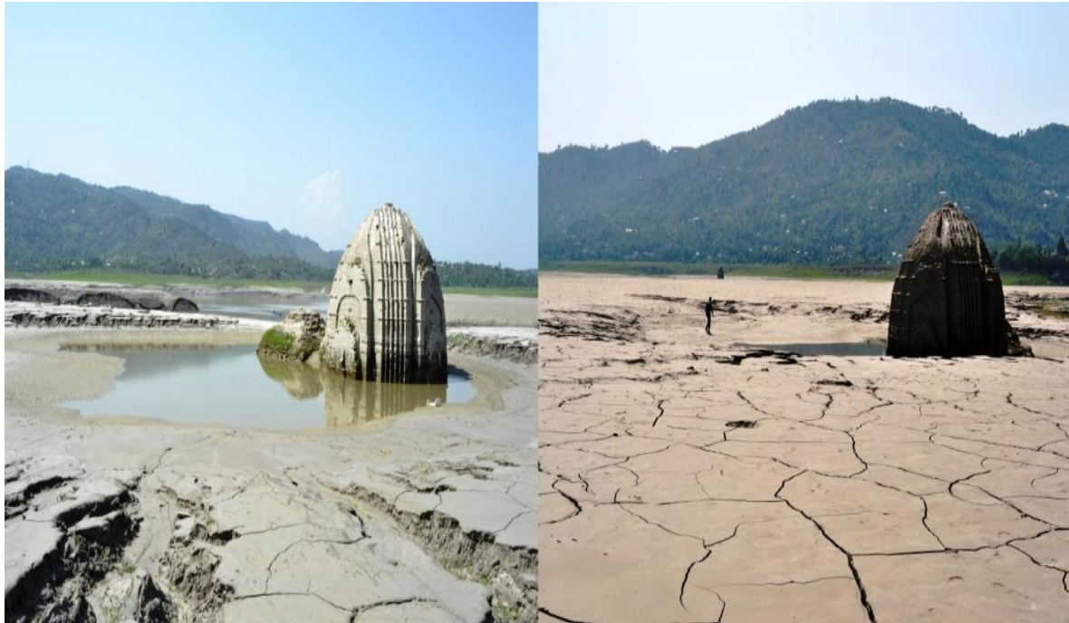
Fig.-4 The Gobind Sagar Lake (HP) is so full of silt that its bed level has raised by at least 5 feet ( http://myboardmyblog.blogspot.in/2011/04/gobind-sagar-submerged-temples.html )
