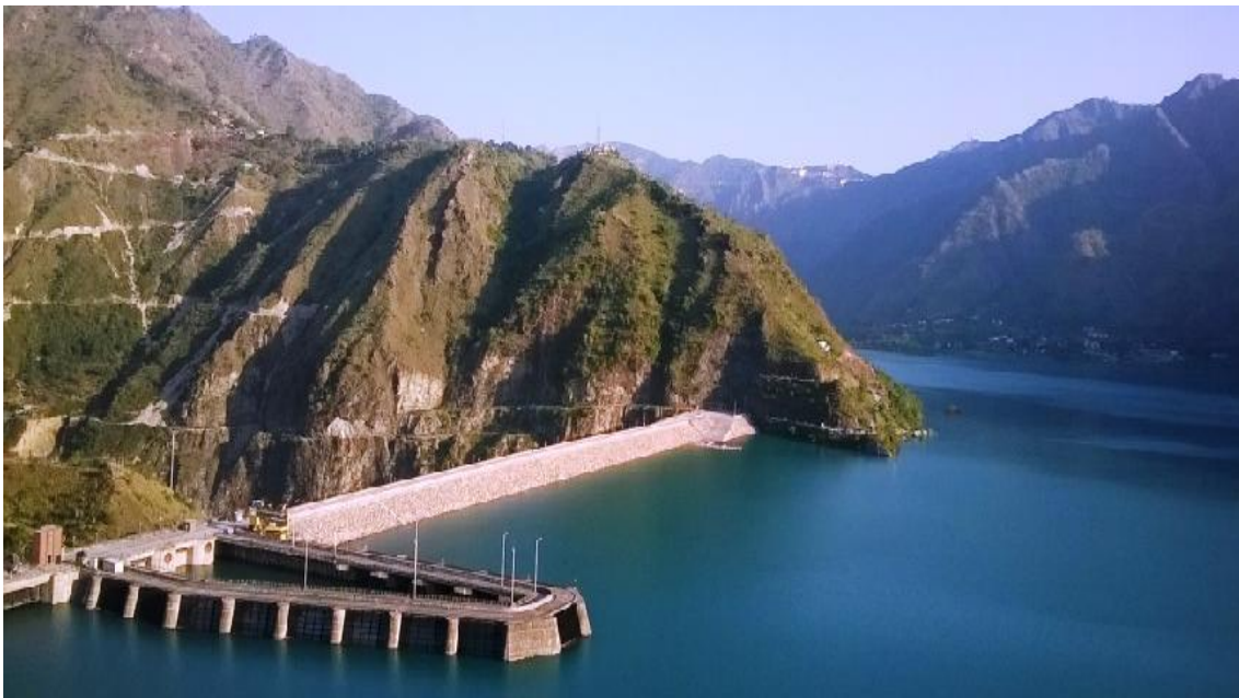
Fig.-12 View of Kol Dam reservoir after completion of project during 2014 (Chand H., Verma K.S. and Kashyap R., Environment Management Plan for Hydropower Project: A
