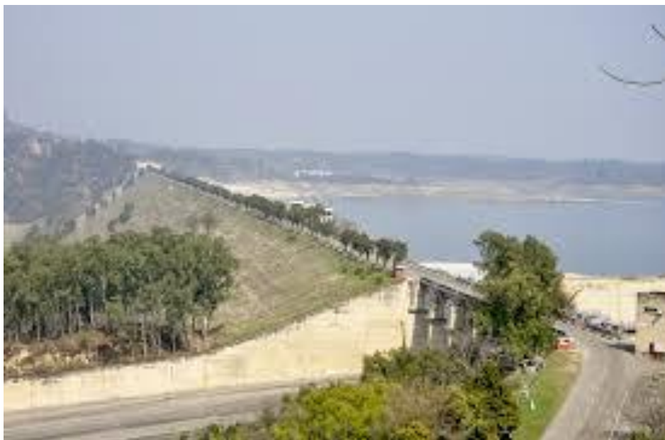
Fig.-11 View of Pong Dam
